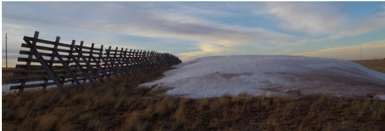
Figure 1. Snowdrift in downstream of the Wyoming type snow fence
