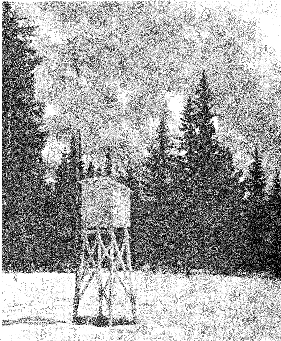
Instrument Shelter on Dark Range Project
