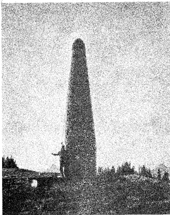
Photo 4. A 26 ft. by 7 ft. radome housing VHF and UHF radio equipment for a trunk drop repeater station.
