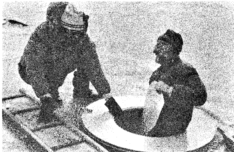
Figure 4. Installing ballast plates used to achieve neutral buoyancy.
